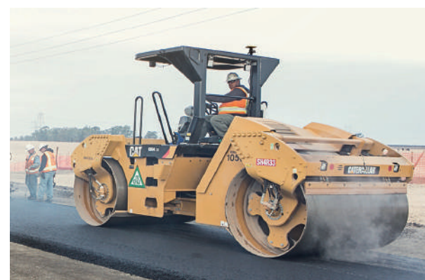
C-53 Intelligent Compaction
